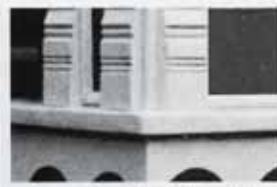
...sanded, nailed, stained or painted.
